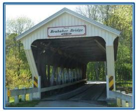
The Brubaker Bridge, built in 1887, can be found on Brubaker Road and crosses Sam's Run Creek. At almost 90 feet in length, the Brubaker Covered Bridge is one of seven remaining Child's truss covered bridges left in the United States. This particular bridge has an open center panel. The Brubaker Bridge is unique because the upper portion of the sides of the bridge have been removed to allow light and a clear line of sight through the bend in the road past the structure.
