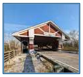
On June 23, 2012, over 100 years since the last covered bridge was built, the all-new Hueston Woods Covered Bridge was dedicated. This bridge is a Burr Arch truss construction, and it has a span of 108 feet over Four Mile Creek in Hueston Woods State Park.
