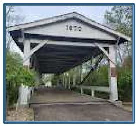
The Germantown Covered Bridge was erected in 1870 and restored in 1963 when it was 93 years old. It is reputed to be the only existing covered bridge of its kind in the world. For 41 years this unique inverted bow string truss covered bridge spanned Little Twin Creek on the Dayton Pike in Germantown, Ohio. In 1911 it was moved to its present location.
